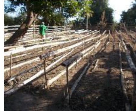
Photo 11: Beroboka North, installation of shade support.
